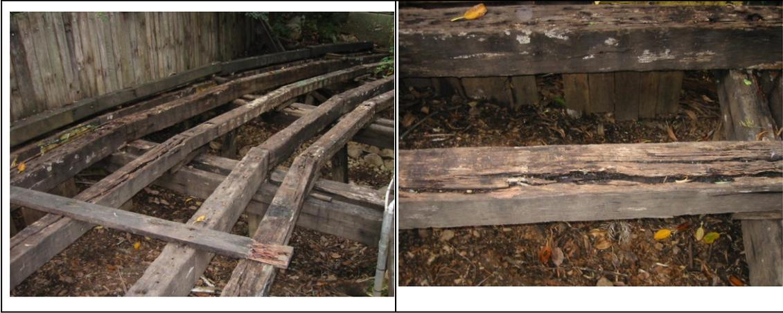
The poor owner of a home in residential subdivision in Brisbane had a rude shock when his timber driveway failed. It was built from recycled timber and would have been very expensive but the timber was worn out before a single tyre passed over it. A situation like this needs the performance, species and grades that we associate with new timber. It will involve limiting the amount of heart in sawn members.
