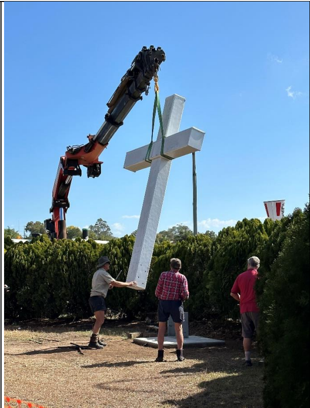
Cross being reinstalled in a steel base.
