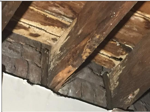
Oregon joists are pristine after 124 years except where there has been moisture entry
