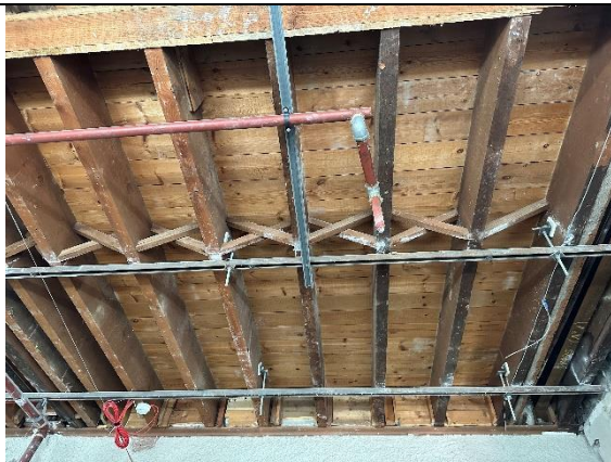
Oregon joists are pristine after 124 years except where there has been moisture entry
