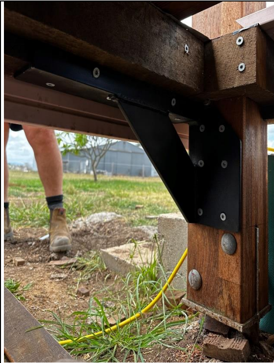
Additional bracing was needed for blade-type post supports.
