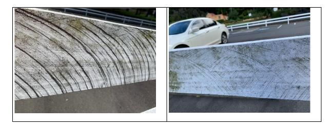
You have to have a fair idea that something is wrong when you see sawing as bad as this. It is not clear in the right-hand image that the angle of the saw marks are running in both directions. It looks as if it was done on a buzz saw on a farm somewhere. So, it would explain what inappropriate material was sold.
