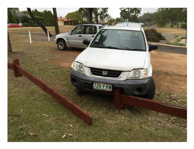
Compare that outcome with these almost 30-year-old traffic barriers I supplied opposite my house. The driver hit the accelerator, not the break (the risk at the above carpark) but the bollard drove the radiator into the motor and stalled the engine. the car was written off with the subframe damage. And it is not designed as a crash barrier!
