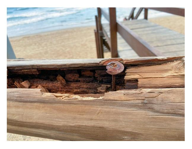
This image shows what can happen when you fasten from the top through poorly treated sapwood or completely untreated heartwood of pine. Fastening from underneath solves all of this.
