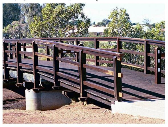
It is not hard to excel at handrails. Here is an example of some of my earlier work. The post is bolted to the joist and a cross transom keeping it rigid and the overhang is no more than 150 mm. (and not a piece of pine in sight.)
