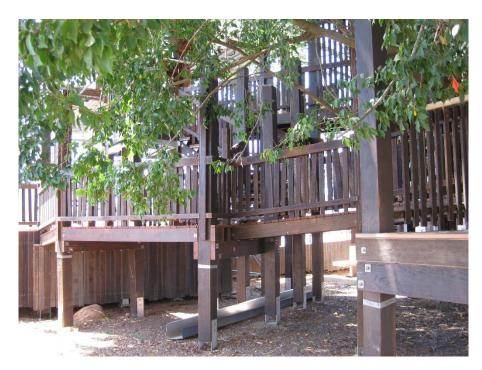
The decks generally follow the advice in this guide for best practice in construction with 120x35 mm decking laid on 75 mm joists with 14# screws installed in a staggered alignment. Posts are installed in stainless steel stirrups and all the fasteners are stainless. The playground is shown during construction in Figure 121 and note the use of conventional fasteners, not tamper resistant.
