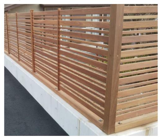
Notice the craftmanship and care in design that has gone into this fence. It is all prefabricated with CNC equipment and there is not the usual back. Both sides are the "front" Notice the quality that it is possible to purchase.
