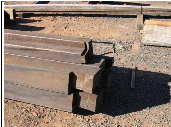
Timber was pre-cut then treated
