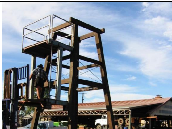
Construction after precutting and treatment
