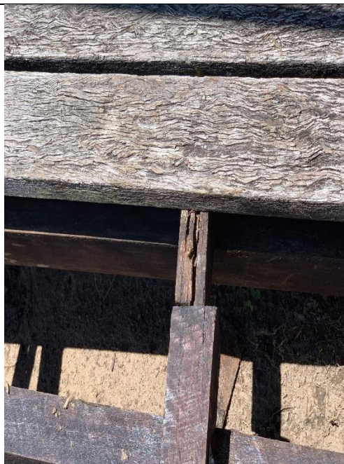
New 75 mm joist against a failed 50 mm
