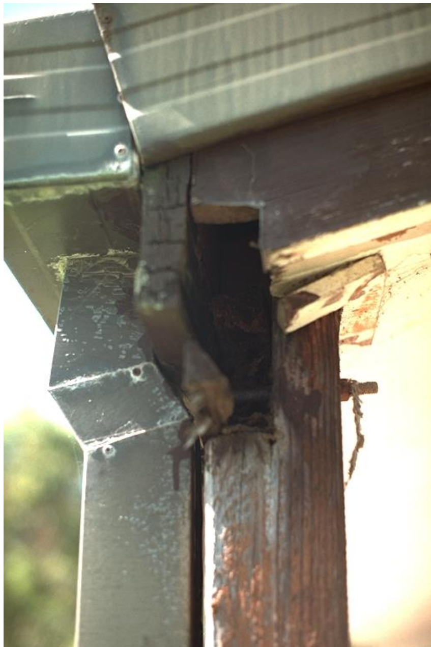
Decaying Oregon verandah roof beam on the Gold Coast
