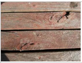
When you stagger and predrill the joist does not The poor quality of decking you may receive if split
