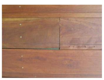
boards and produce dressed products from it and prepare yourself a claim. The image to the right shows recycled spotted gum which has shrunk so badly it that the shiplap is no longer lapping and you can see the insulation underneath.
