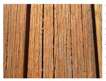
The picture to the left is of 13 year old blackbutt used in a barbecue table in full sun. It is not aging gracefully. When you go away from the timbers that were traditionally used in an application and just go by a durability rating you can get this disappointing result. When writing to one timber merchant in Perth recently about jarrah, he commented "It's funny you mention Colour, over here lighter wood preforms miserably in our climate,
