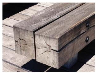
Firstly what is right with this design is that it is not bolted through the top allowing moisture into the heart. That can cause early degrade.
