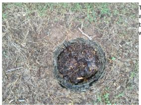
These bollards are not capped and it is only when they get some age on them that the need for caps becomes obvious. The band of treated sapwood is in good shape but the centre, which will nor accept treatment is deteriorating.
