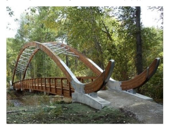
The B**ow Bridge** on Big Wood River \_ Draper, ID - 160' x 6' Pinned Arch Timber Bridge, which crosses the Big Wood River at the Draper Preserve in Hailey. The Bow Bridge of the Big Wood River was designed to mimic a recurve bow that appears to have been dropped from the sky, landing string side down. The bridge now connects the East and West banks of the Big Wood.
