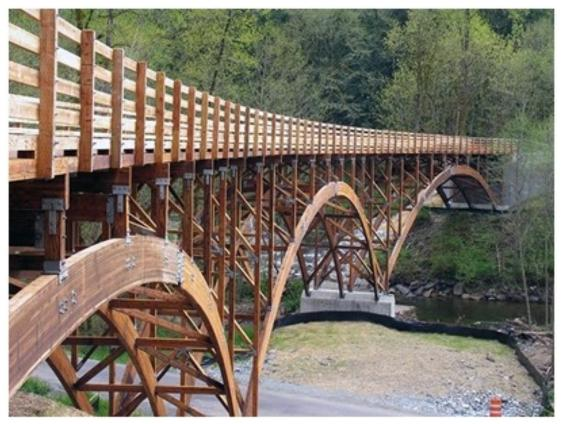
The Lower Burnett Road Bridge is a three-span, timber arch bridge in Buckley,
