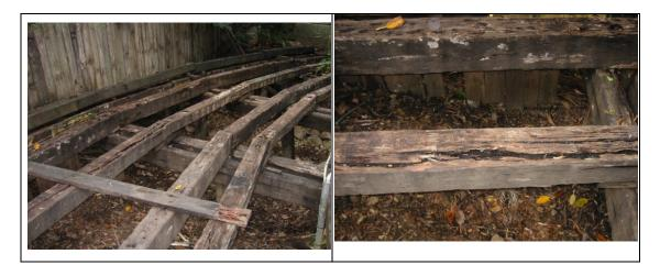
The poor owner of a home in residential subdivision in Brisbane had a rude shock when his timber driveway failed. It was built from recycled timber and would have been very expensive but the timber was worn out before a single tyre passed over it. A situation like this needs the performance, species and grades that we associate with new timber. It will involve limiting the amount of heart in sawn members.
