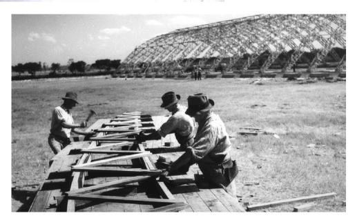
The smaller Australian hangars were built from lineal 100x50 and simply nailed together yet the technology used in them was ground breaking and utilised timber up three times more efficiently than it had been before. The connections had to be much better.
