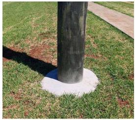
A reader recently sent me this image commenting that whoever put this post in does not read my newsletters. Hardwood and concrete do not mix. I have seen ironbark rot of at groundline in 14 years when set in concrete. Remember, use natural earth if suitable, fine crushed rock or no fines concrete. This is one of my <u>Seven Deadly Sins</u>. So, seeing how easy it is to go wrong with a timber post, wouldn't it be better to use steel?
