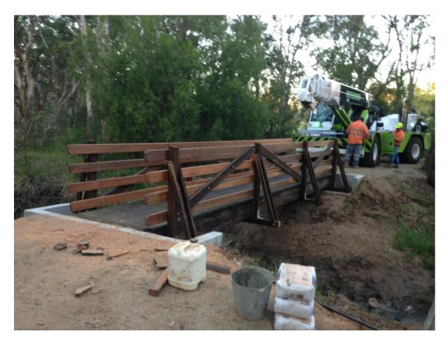
The cost of timber girders has risen so much, and their availability is getting so poor that it is almost better to go straight to steel. This is unfortunate as a well built log bridge is very durable bridges with minimal issues, especially when you do the abutments correctly.
